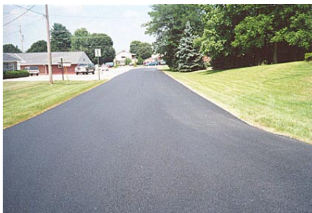
Figure 4. The reclaimed road after paving
