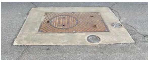
Manhole restoration to surface
