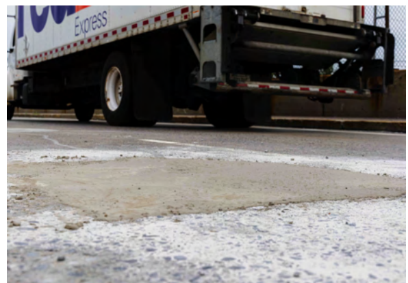
New York State DOT bridge deck repairs
