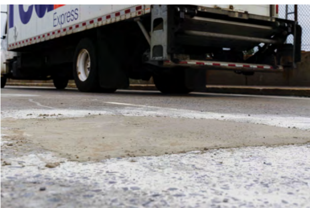
New York State DOT Bridge Deck Repairs
