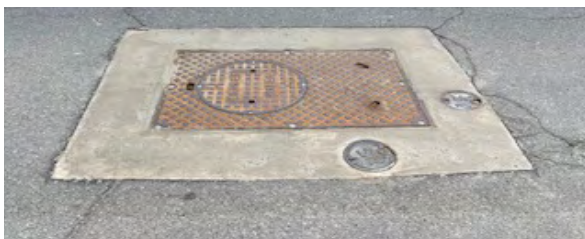
Manhole restoration to surface
