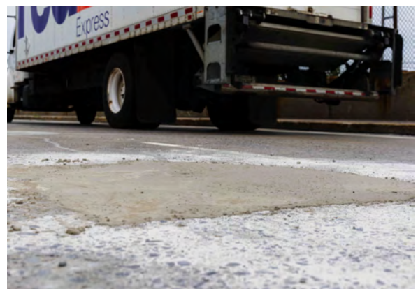
New York State DOT bridge deck repairs
