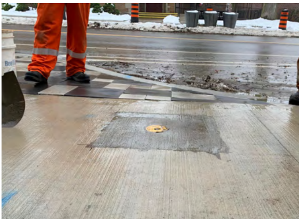
Gas valve box in sidewalk
